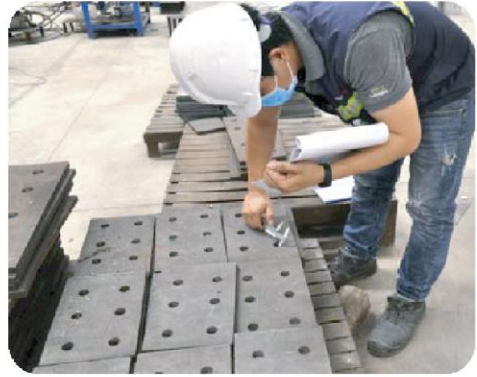
DRILLING & CUTTING CHECKING
