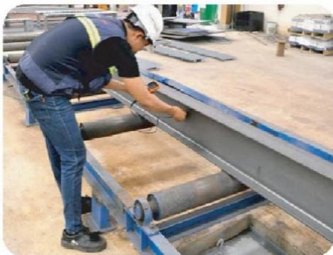
SHOT BLASTING CHECKING
