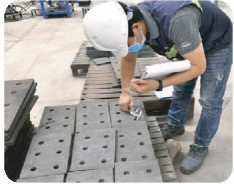
DRILLING & CUTTING CHECKING
